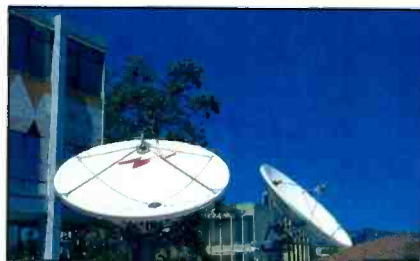
Although fiber plays a large role in how signals are handled, two dual-band TVRO dishes are required for some program acquisition.
